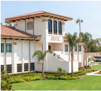
HEATH ACADEMIC CENTER EXTERIOR IMPROVEMENTS $200,000
